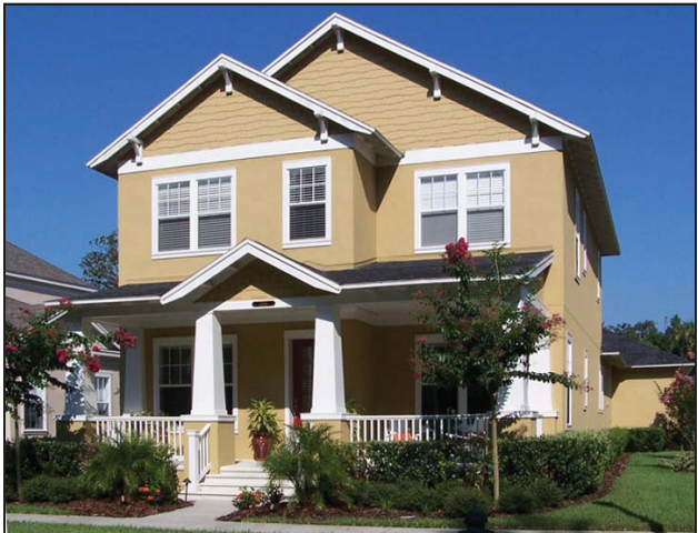
This home displays several characteristics of the Craftsmen style including exposed rafter tails, tapered columns on square bases and brackets roof overhangs.
