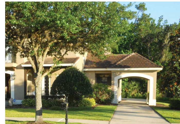
A porte cochere helps to mitigate the impact of the driveway on the street.
