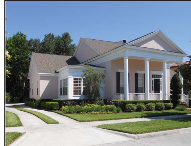
This Classical style house features a temple front with classically proportioned columns and pediment which dominate the front facade.
