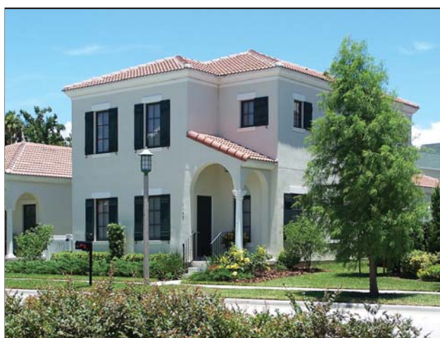
While simple in massing and detail, the barrel tile roof, casement windows and smooth stucco finish clearly describe the Mediterranean style.
