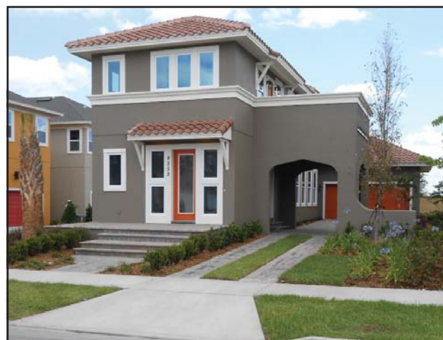
The arched porte cochere helps mitigate the street garage access of this Transitional home.
