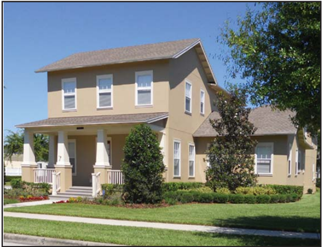
This craftsman home has the main roof structure parallel to the street versus the home below with the main roof structure perpendicular to the street.
