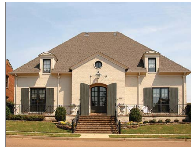
Painted brick is an appropriate alternative to stucco on this perfectly symmetrical European Vernacular home
