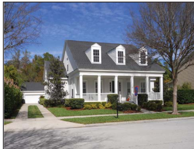
Simplified dormer, porch and eave details contribute to the quality of this Southern Vernacular home.
